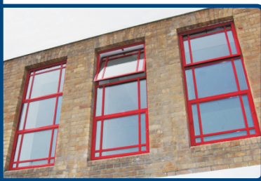
W20 replica replacement polyester powder coated and double glazed steel windows with true steel glazing bars
